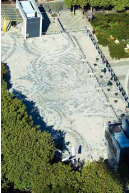
FISHER PAVILION ROOF
