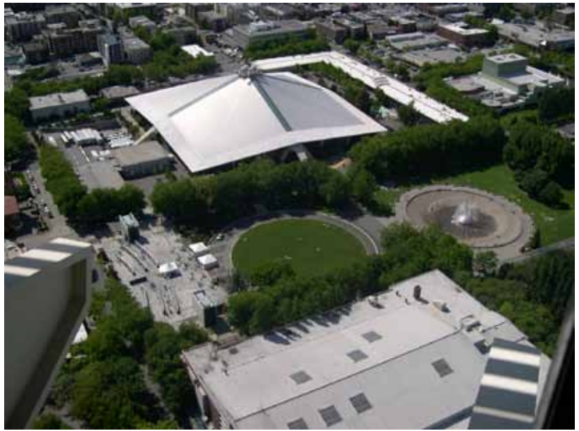
OVERHEAD OF FOUNTAIN & KEYARENA
